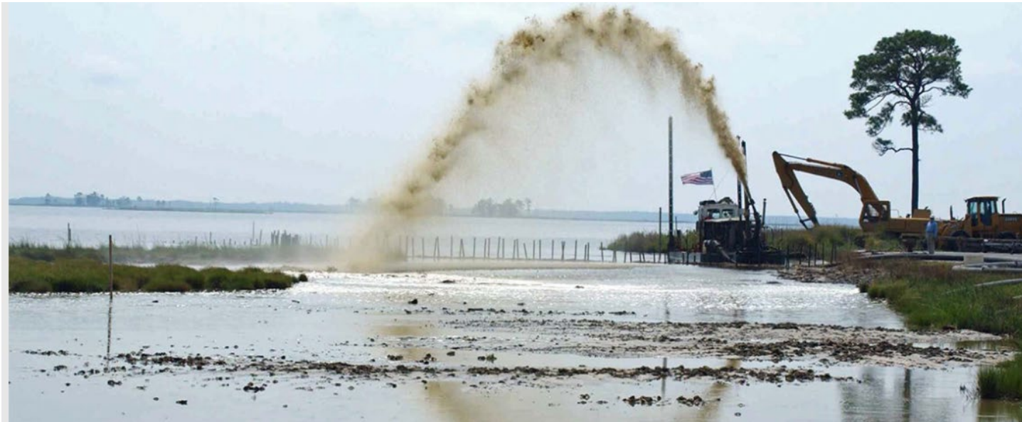
Thin layer placement of dredge spoil material into a marsh area to preserve marsh habitat due to sea level rise
