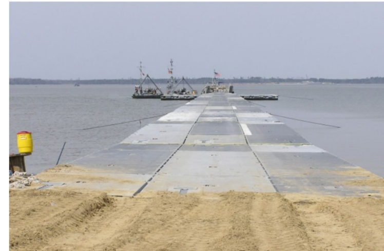
A modular floating pier set up for training on JBLE-Eustis. These piers are used for ship to shore delivery of supplies in real-world operations.
